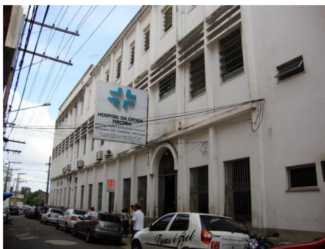
Figura 13- Fachada principal do hospital
